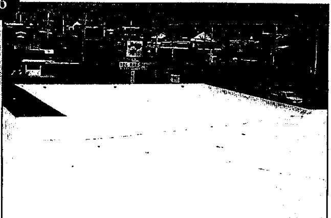
After/Top Coat: White, highly reflective acrylic top coat is applied over the base coat.
