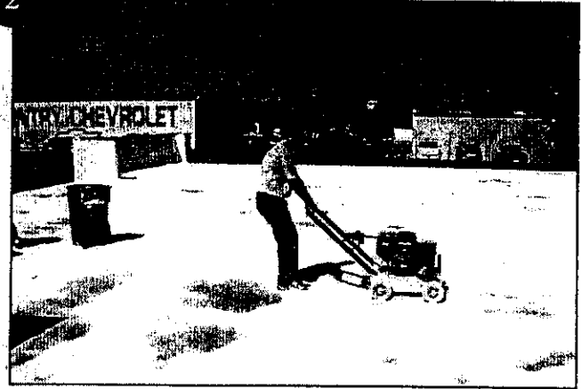
Surface Preparation-Scarifying: Existing foam roofs can be scarified before the foam is applied.
